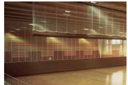
Mesh-synthetic leather combinations are usually used as room dividers in large halls so as not to impair the ingress of daylight and the visual size of the hall. There is no noise separation when room dividers are used.
