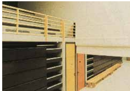
Partition cut-outs are needed for handrails or steps in the area of the dividing curtain.
