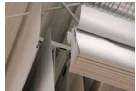
Blinds and partitions to exclude extraneous sound in the roof area when acoustic demands are high.
